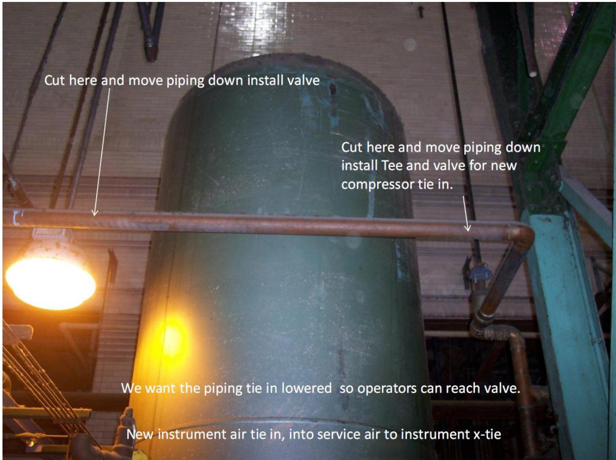
Cut here and move piping down install valve
