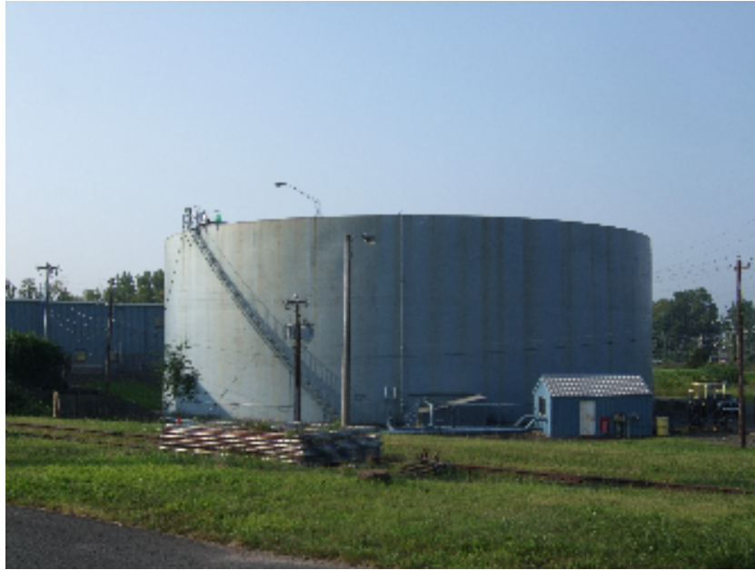
Photo 1: General View of Tank 6
