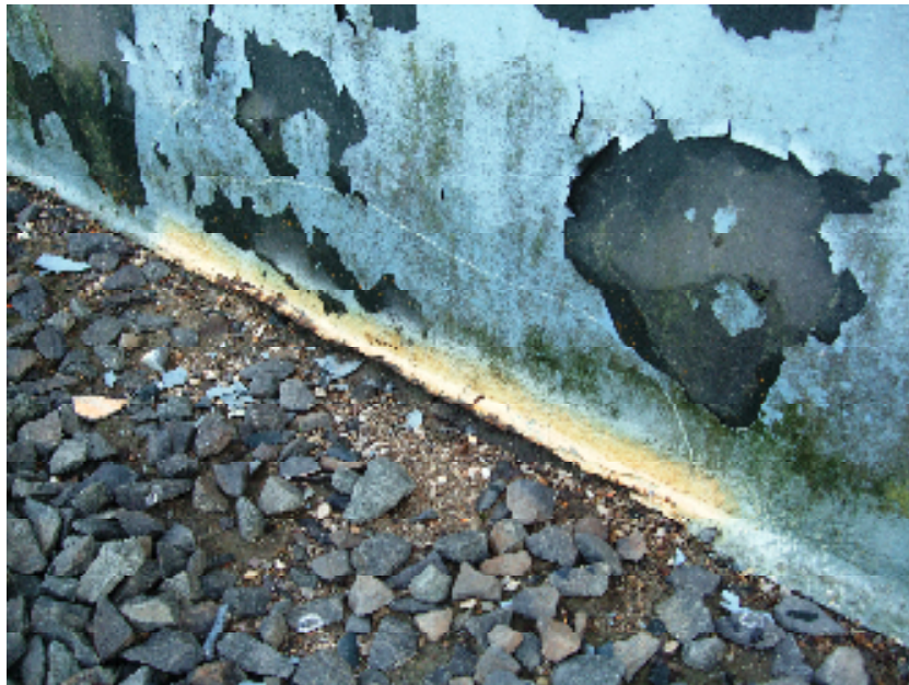
Photo 2: Area of Most Severe Chime Corrosion (west side of tank)
