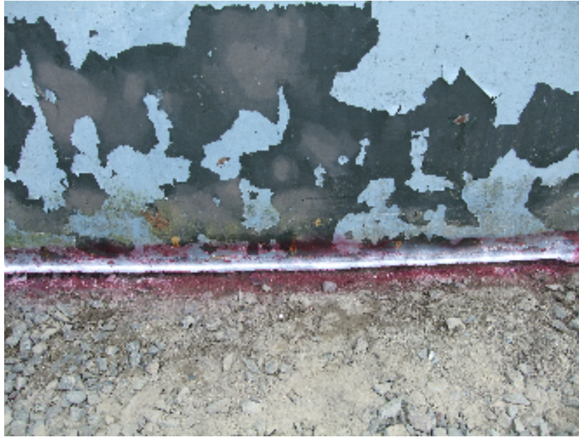
Photo 3: Results of Dye Penetrant Examination (Note absence of linear indications)
