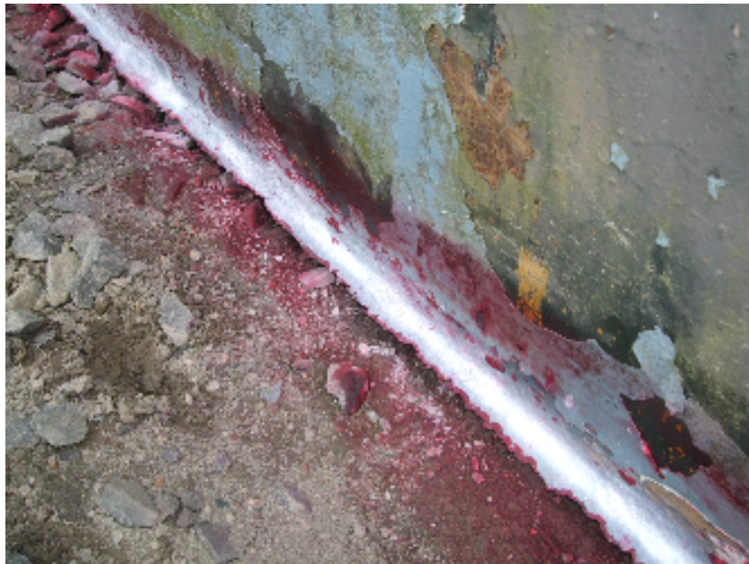
Photo 4: Close-up View of Dye Penetrant Inspection
