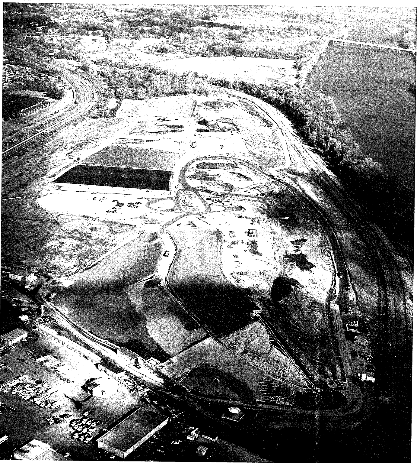
Hartford Landfill Final Cap Installation in Progress
