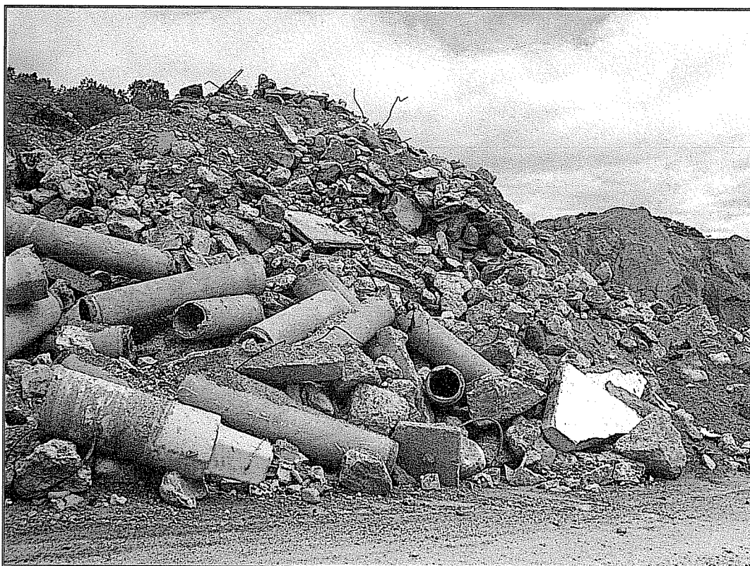
Photograph of typical concrete staging pile to be processed on Area B of the site, facing west-northwest.
