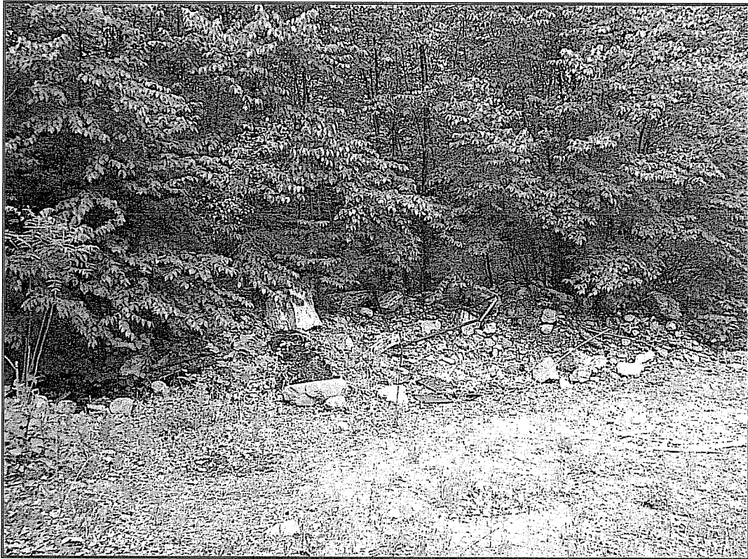
Photograph of base of borrow pit on Area C of the site, facing west.
